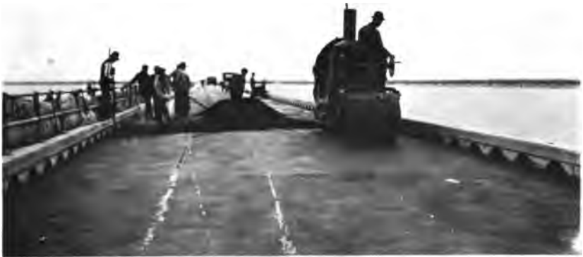
Surfacing the Yolo Causeway.
